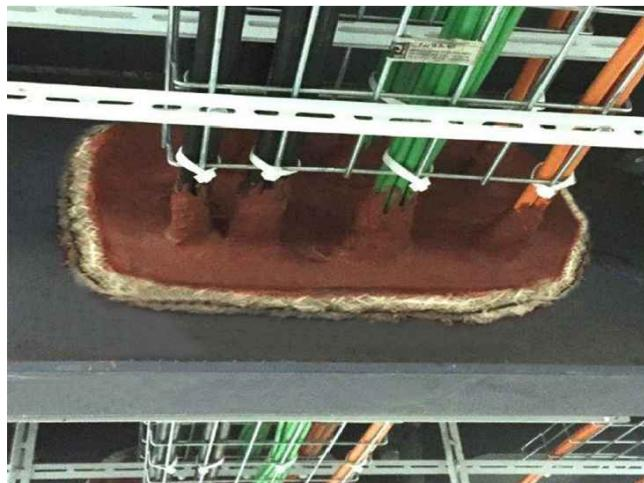
Class A fire protection system on bulkhead (MED NR.288119CS/001) penetration through electric cable according to IMO Res. MSC. 307(88)-(2010 FTP Code) - IMO MSC.1/Circ. 1488
